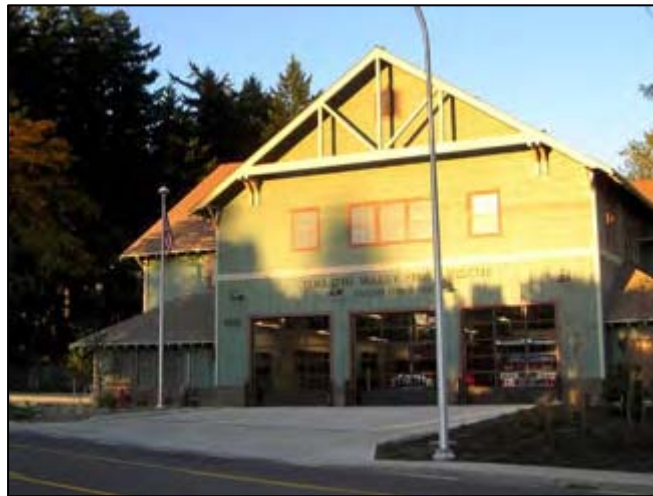
TVF&R Fire Station No. 53
